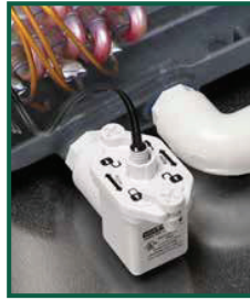
Auxiliary Port on Primary Drain: SS2
