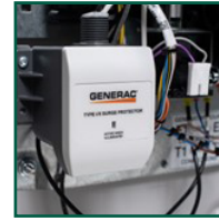
Integrated Surge Protection on 100-200amp Switches
